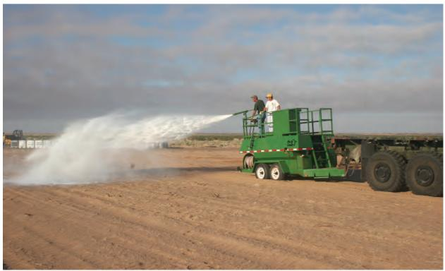
Photo 17. Spraying helipad with dust palliative using tower gun on Easy Lawn hydroseeder
