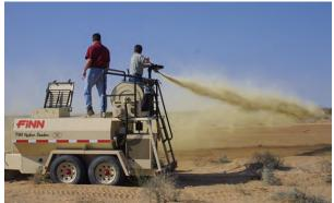
Photo 6. Distributing emulsion onto helipad using tower gun
