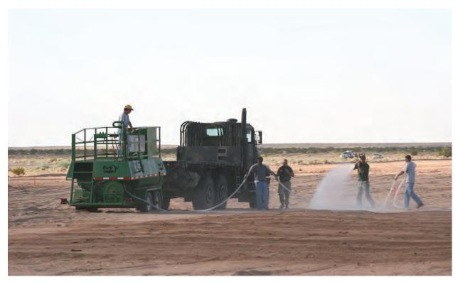
Photo 16. Treating helipad using hand-held hose on Easy Lawn hydroseeder
