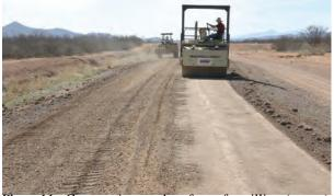
Photo 11. Compacting road surface after tilling (step g)
