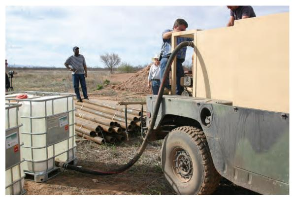
Photo 32. Transferring dust palliative from 275-gal shipping container
