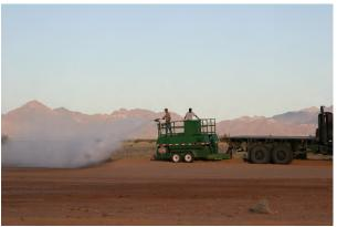
Photo 2. Spraying helipad using tower gun (step *d*)
